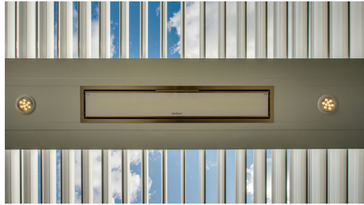
Beam Chases (Can Lights, Sonance Speakers etc.)
